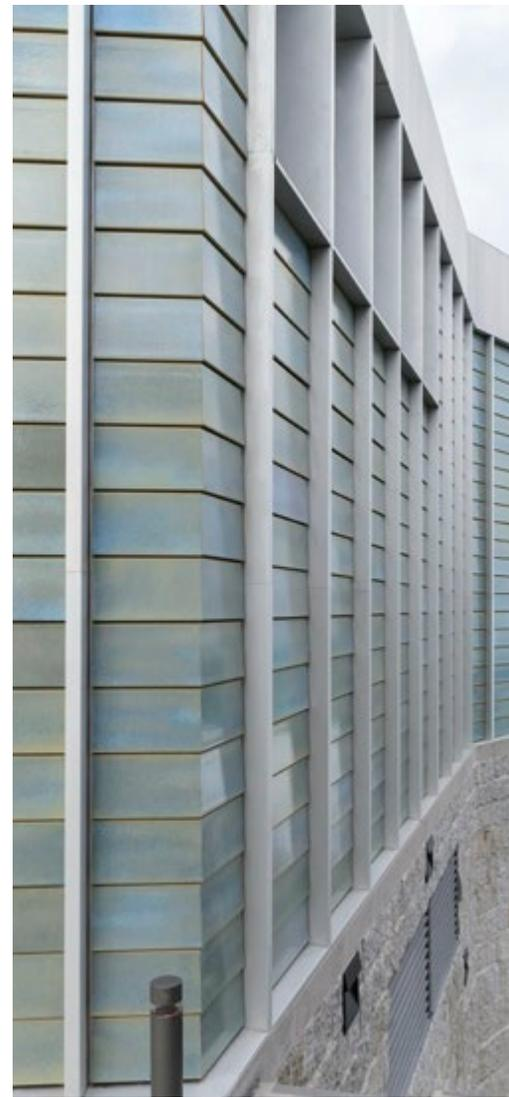
Meanwhile, back at **City Village** the tallest of the four volumes on the scheme that rises above the city – a 20-storey tower – is at once designed to stand out and disappear by being designed with the same cladding composition as the other terracotta elements, but carried out in a high-gloss light blue terracotta tile. The tower reflects the colors of the cityscape and sky, giving the project an unexpected lightness.
