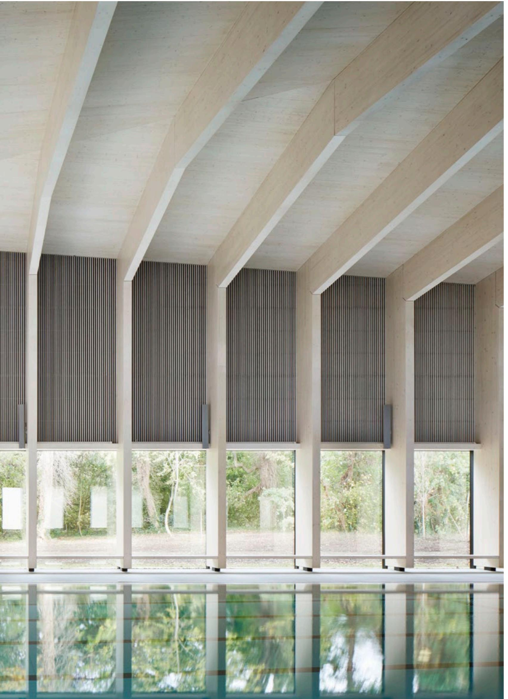
vertical ribs helps to meld the building and landscape. Standing seam cladding is utilised because it is a more traditional form of construction, which responds to key features of the listed Main House. The deep columns of the all-timber construction and wrap-around glazing, which afford direct views from the water into the woodland, give the sense of swimming amongst the trees.'
